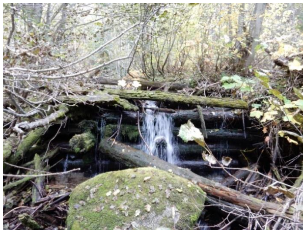
Photo 1. Looking upstream at a remnant of a log crib structure that spanned the north fork valley bottom. This structure appears to have been used as a retention dam to supply water to the flume system.
